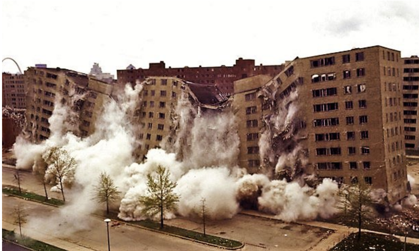
Minoru Yamasaki, Pruitt-Igoe Housing, St Louis, 1972 demolition
