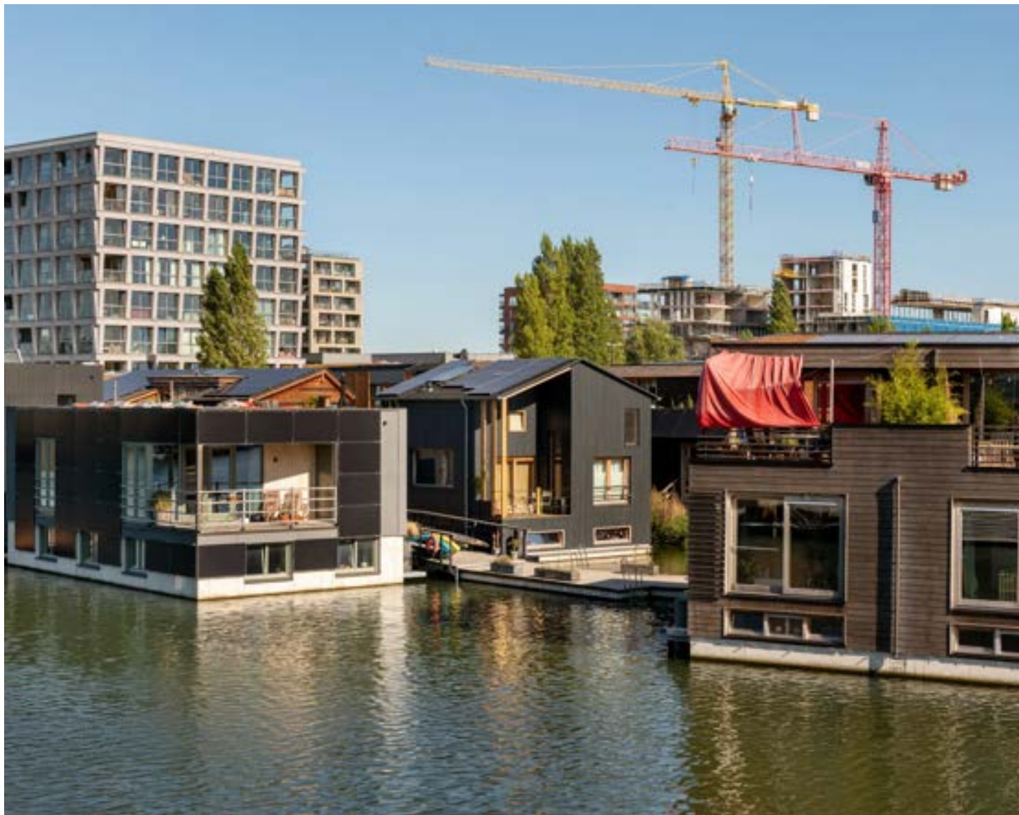
The residents of Schoonschip chose their own construction materials, but most built houses with timber frames and insulated them with materials like burlap or straw. Max Pinckers for The New York Times
