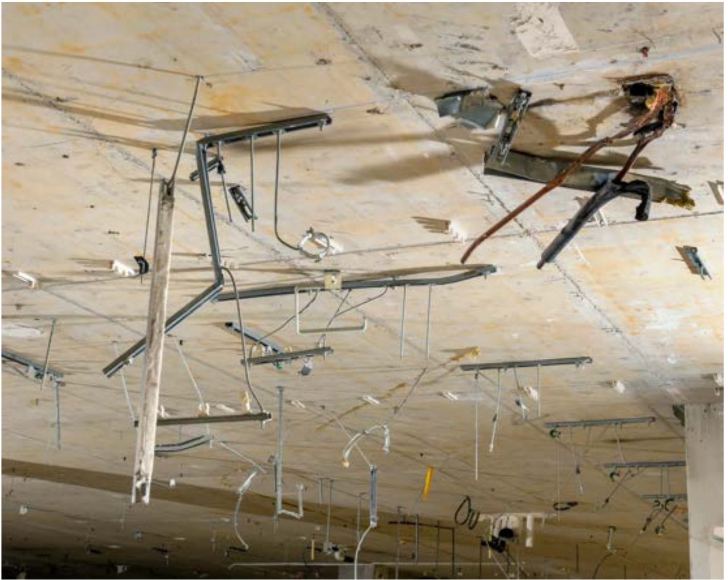
New Horizon plucked electronics, fire safety equipment, wood and aluminum from the hospital for reuse. It also has plans to recycle the concrete. Max Pinckers for The New York Times
