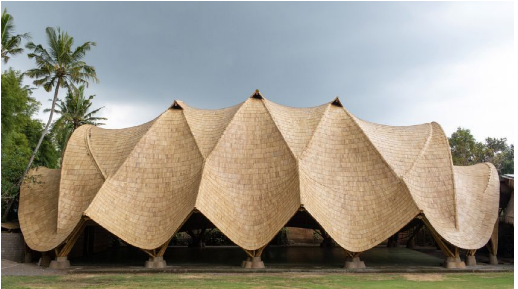
Ibuku, Arc Gymnasium, The Green School, Bali, 2021
