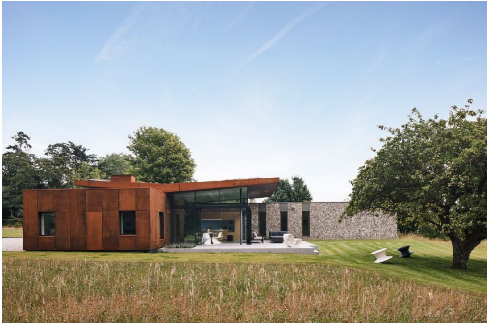
Hudson Architects, Coast House, Norfolk, UK, 2022
