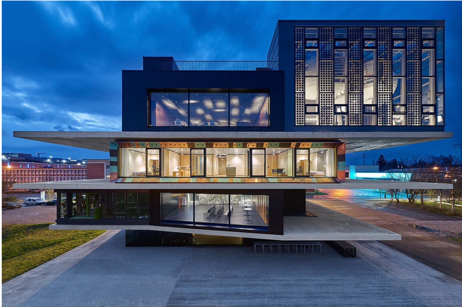
Werner Sobek, Urban Mining and Recycling Residential Unit, Dübendorf, Switzerland, 2018
