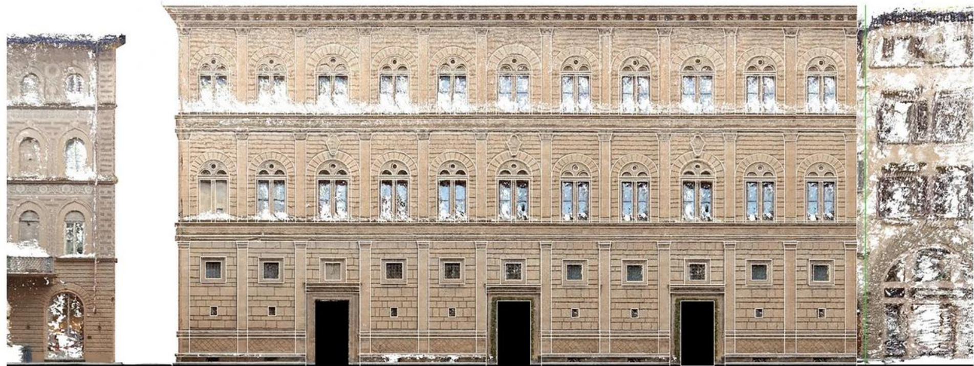
Façade Reconstruction 11-bays
